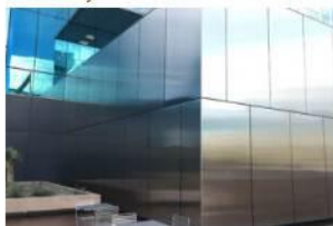
Building exterior insulation wall panels
