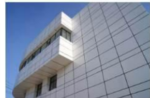
Building wall panels.
